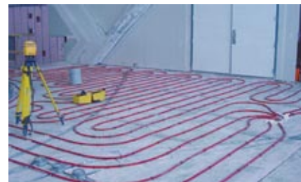
ECB beneath PVC tubing laid for a hydronically heated floor.
