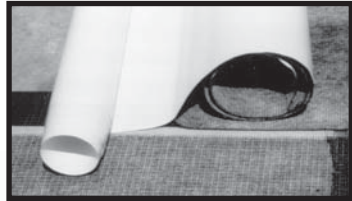
OVERLAP: Strataflex side seams. Remove film from 2" double-stick edge on underlying sheet and carefully press into place.
